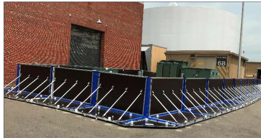
Test deployment of temporary flood barriers Electrical Telecom Building at Logan
