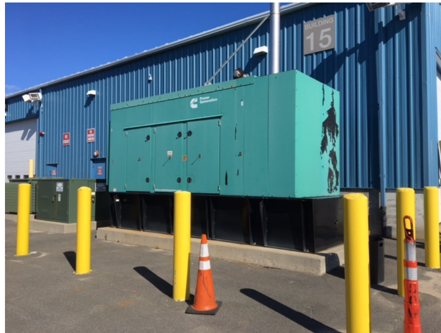
Elevated Platform at CTDFC
