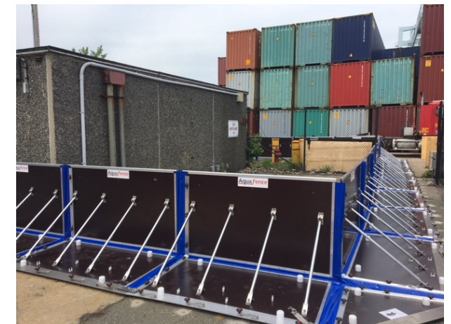
Conley Terminal test deployment
